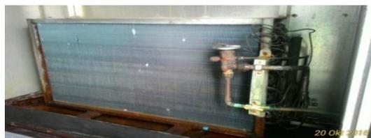
Gambar 4.7: Koil Pendingin (*Cooling Coil*)
